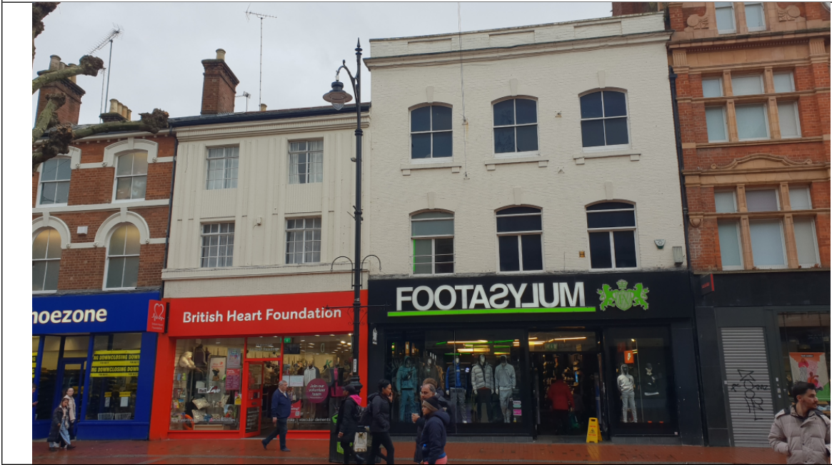
Fig. 3: 84 Broad Street. Source: RBC Photo, February 2023.
