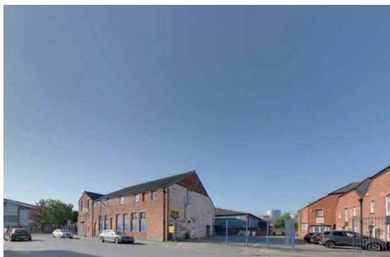
Existing view from Northfield Road
